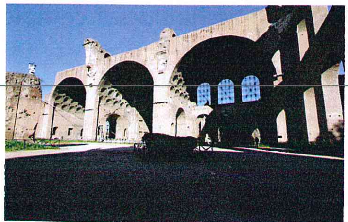
Fig. 23 – An internal view of the monument with structural reinforcements installed.
