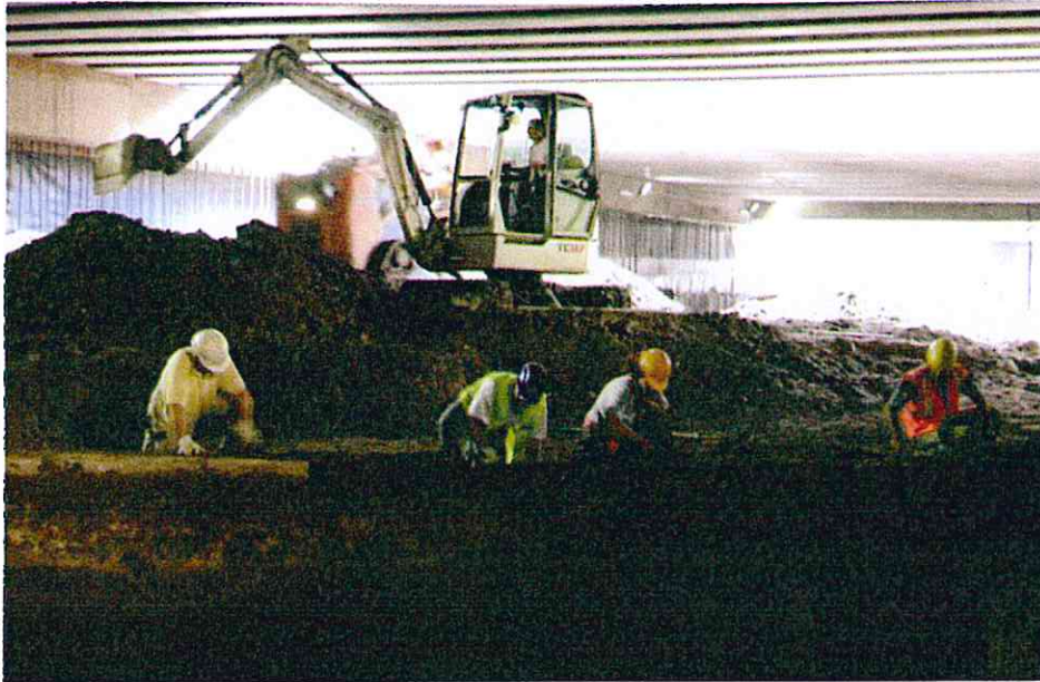
Fig. 2 – Archaeological excavation during the construction of the station (top-down method).
