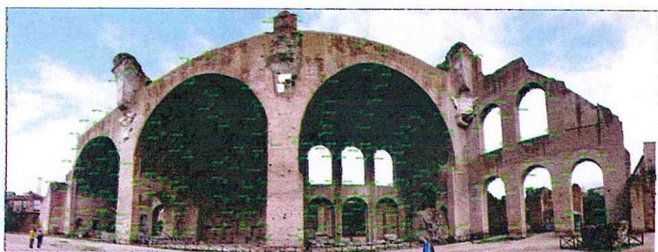
Fig. 25 - An internal view of the monument with the monitoring instrumentation installed.
