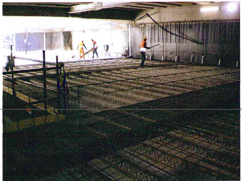
Fig. 7 – The construction of an horizontal floor with self-bearing prefabricated.
