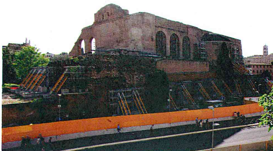
Fig. 24 - An external view of the monument with the temporary supports installed.
