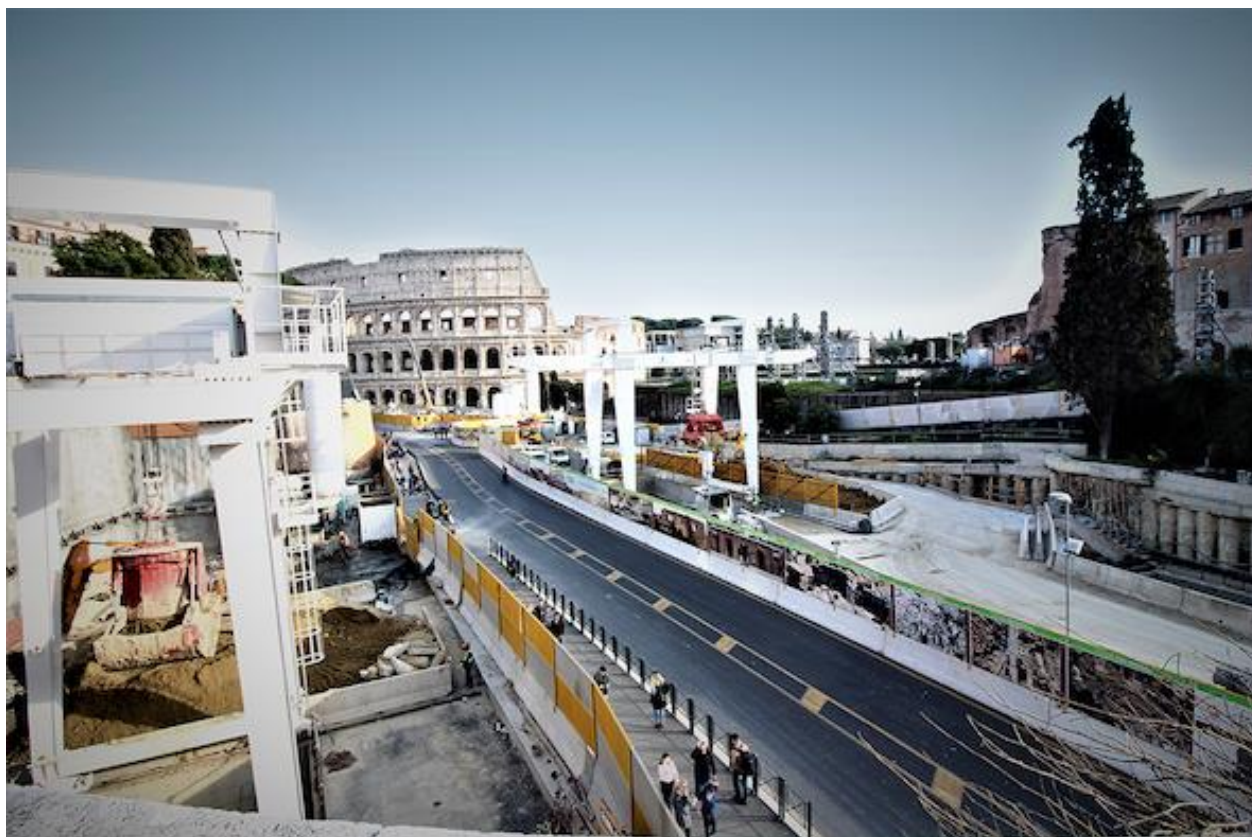
Roma, Fori Imperiali station - Courtesy World Tunnel Congress
