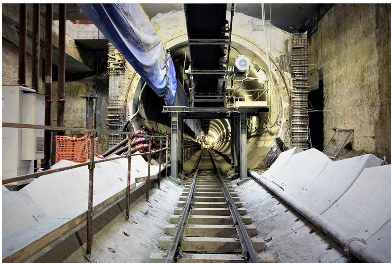
Roma, Amba Aradam-Ipponio station TBM tunnels – Courtesy World Tunnel Congress
